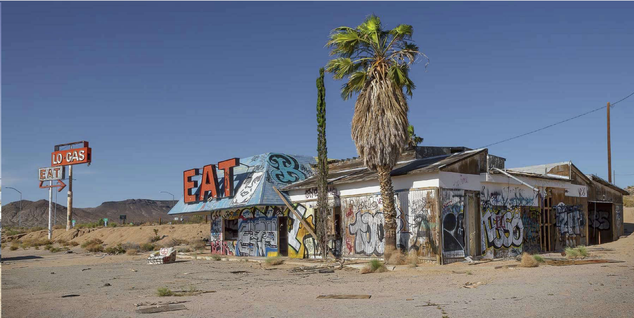
Abandoned Restuarant, Along I-15, Exit 259, California - 2023
